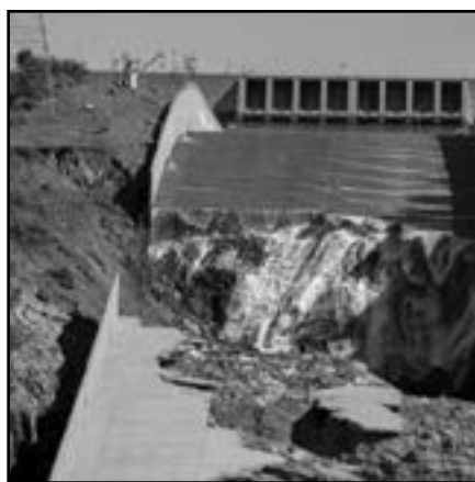
Halfway down the Oroville Dam spillway a massive crater attests to the power of water and gravity. Photo credit: Feb. 27, 2017/ Dale Kolke / California Department of Water Resources
