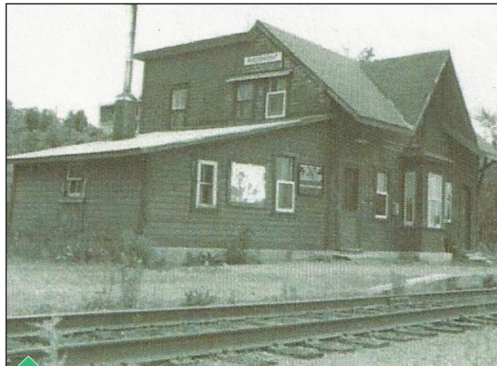
The Piedmont old train station
